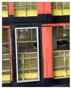
Creating a watertight and airtight seal with certified fire resistance, the ARBOSHIELD Pro® EPAM connects a concrete structural frame or steel frame to SFS sections and exceeds the current Building Regulation and Approved Document B requirements for a fire and weathertight seal that bonds even in -40°C temperatures, futureproofing the project.
