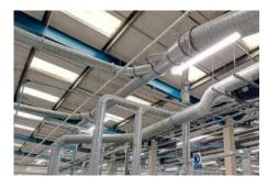
System upgrades included replacing and extending ducting, adjusting diameters to optimise waste flow velocities, and installing Paramount Shoe diverters throughout. This allowed for waste segregation, enhancing returns on waste and assisting customer's sustainability targets.
