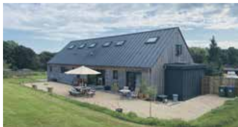
A family house built with naturally insulated passive panels (NIPPs) constructed to passive levels of airtightness and energy efficiency, the complete construction is made using natural and sustainable materials. Image courtesy of Kithurst Builders.
