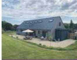
A family house built with naturally insulated passive panels (NIPPs) constructed to passive levels of airtightness and energy efficiency, the complete construction is made using natural and sustainable materials. Image courtesy of Kithurst Builders.
