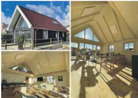
The COP 26 House co-sponsored by Ecomerchant and built for the Glasgow COP is an all-timber construction with no steel, concrete or plastics used in its construction. Insulation is Steico wood fibre, heating by Herschel infrared panels. The COP26 House beats the RIBA 2030 Challenge carbon target by a substantial 22%
