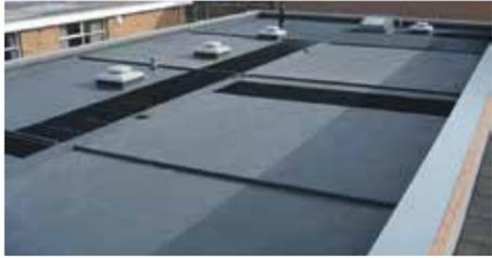
Tuff Waterproofing is a provider of waterproofing liquid solutions for flat roofs, which are comprised of GRP, flexible GRP and polyurethane. Using its advanced TuffStuff® formula range, which uses the latest liquid polyester resins, glass fibre mat reinforcement and flexible edge trims, it creates a fully integrated 100% waterproof seamless finish. The TuffStuff® product range is used for various applications and across multiple domestic and commercial environments.
