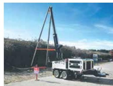
treatment systems. All our boreholes are constructed using the cable-tool percussion method - preferred by the Environment Agency (EA) when drilling the chalk aquifer – and are logged with the BGS. Our underpinning ethic is that we want to protect the aquifers from which we make our living.
