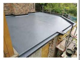
uffStuff® has created the best multipurpose GRP roofing system on the market, with its TuffStuff® Flexible GRP already receiving rave reviews from customers. One resin with endless possibilities, the Flexible GRP provides an exceptional combination of versatility and durability. Quick to lay, with no need to strip or re-deck a roof, this fast-curing system saves time and money.
